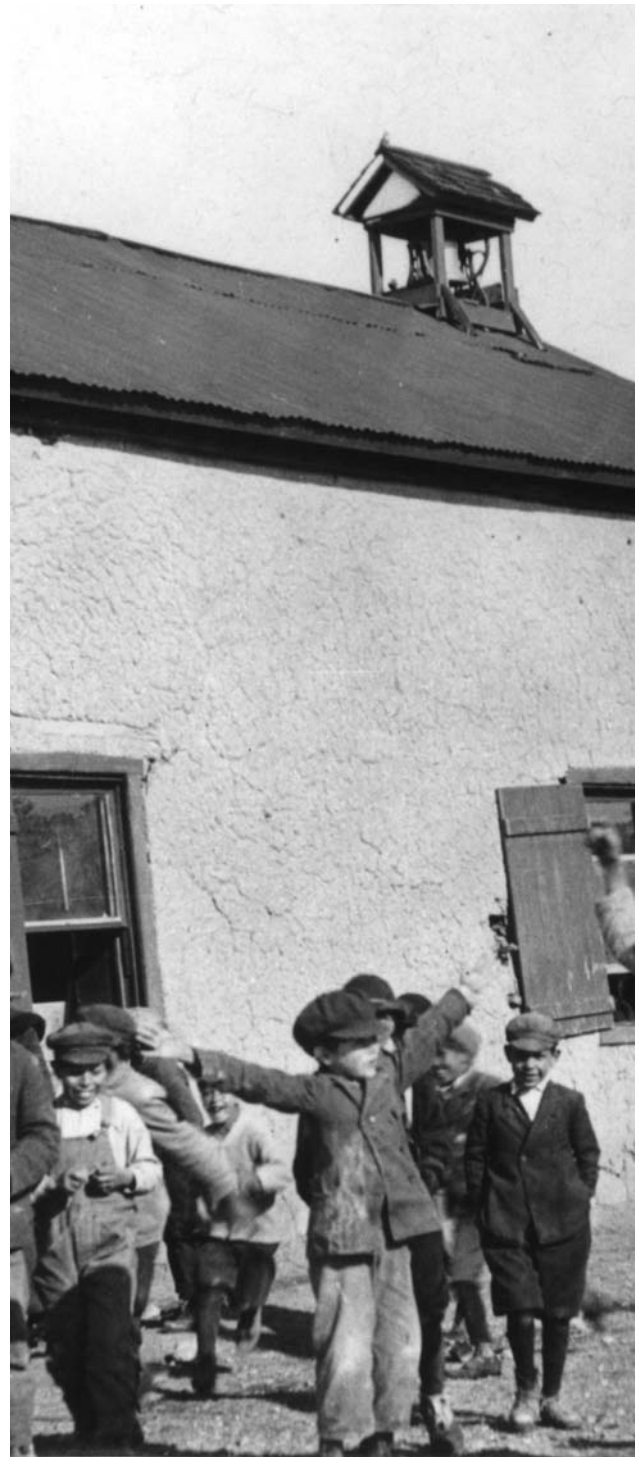
Children at the Picacho Village School in Lincoln County, 1915. By retrofitting older school buildings and implementing energy efficiency practices, more of New Mexico's education dollars can reach the children. Photo courtesy Museum of New Mexico, #1374.
