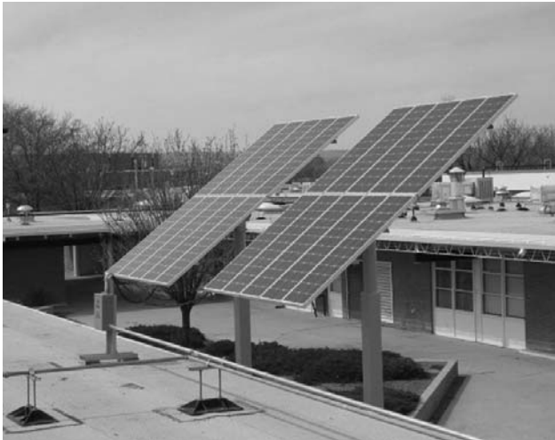
One of the first projects of the Schools with Sol initiative, this 1-kilowatt solar photovoltaic energy system at Rio Grande High School in Albuquerque will produce hot water and electricity and help reduce the school's energy costs. Photo by Brian Johnson, used by permission of The Sacred Power Corporation.
