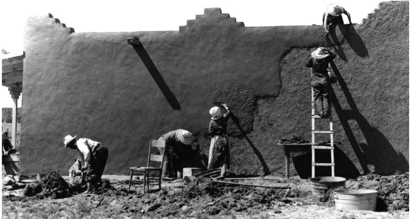
Plastering a house in Chamisal, 1940. Photo by Russell Lee, courtesy the Library of Congress, LC-USF 34-37082.
