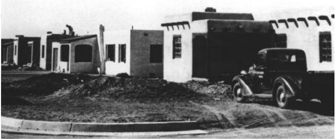
Tax incentives and subsidies are often used to promote economic development and job creation, like the construction shown here in Albuquerque in 1942. Courtesy Palace of the Governors Photo Archives (NMHM/DCA), #183307.
