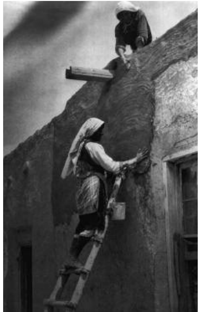
Women plastering an adobe home in Paguete, New Mexico, near Laguna Pueblo, 1925. Photo by Edward S. Curtis, Courtesy Library of Congress, #LC-USZ62-80166.
